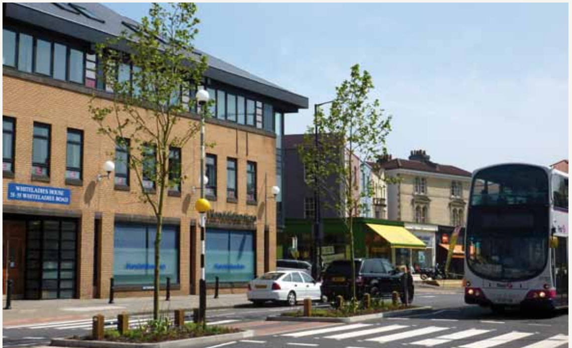
The creation of a central reserve with trees along Whiteladies Road demonstrates how green and grey infrastructure is being combined in Bristol to deliver a better local transport system. © TreeBristol
