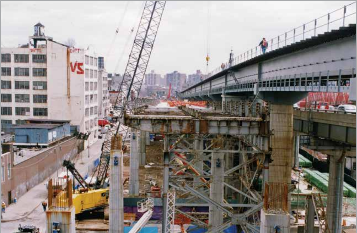
Williamsburg Bridge reconstruction in the 1990s
